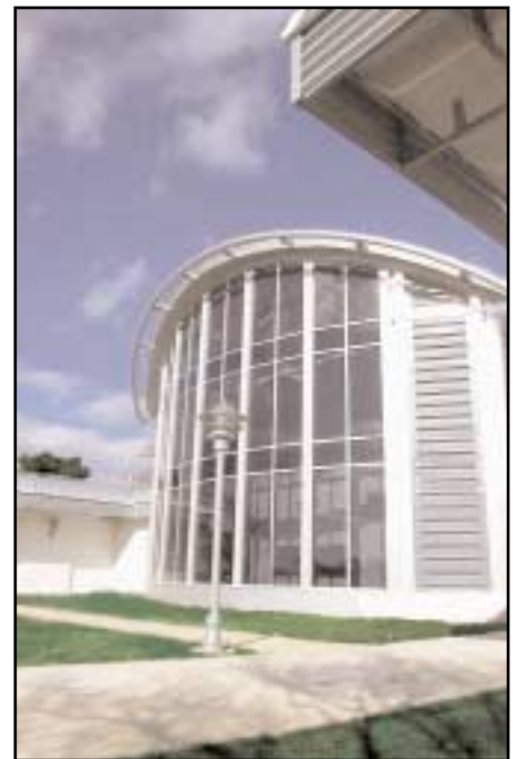
Advanced Manufacturing Processes Lab
